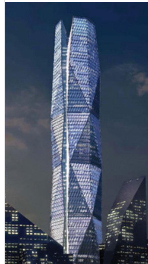
Capital Market Authority Tower
